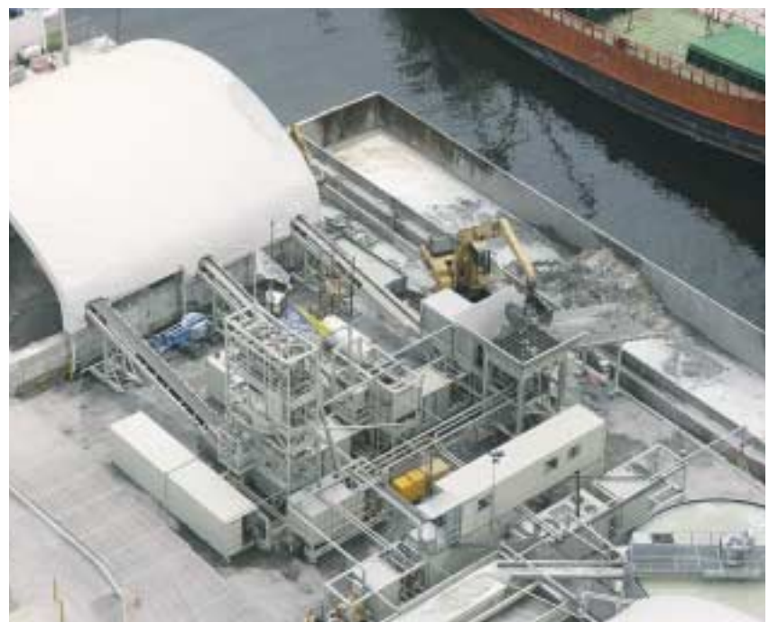
MSWP at Miami River deepening project, USA
