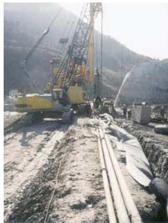
Installation Geolock system, Korea
