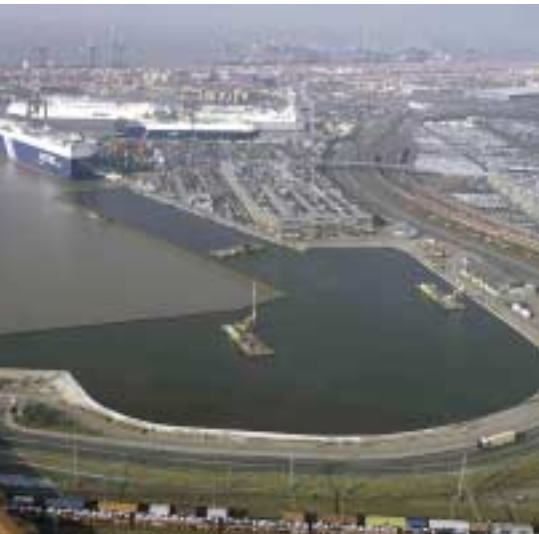
Installation BeauDrain-S system silt depot Bremerhafen, Germany
