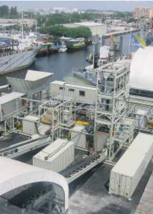
MSWP at Miami River deepening project, USA
