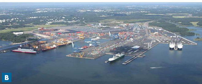
A View of the AP jetty.
